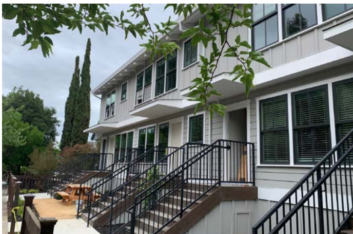
147 Ross Street Apartment building renovation is nearly complete.
