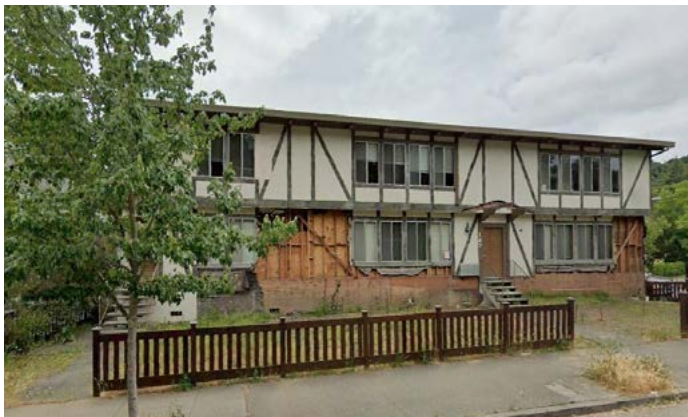
147 Ross Street Apartment building before renovation.
